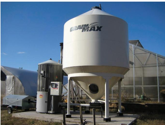
**Figure 4.** This commercial-sized pellet boiler is equipped with a storage bin and an ash cart, part of the automatic ash removal system.
