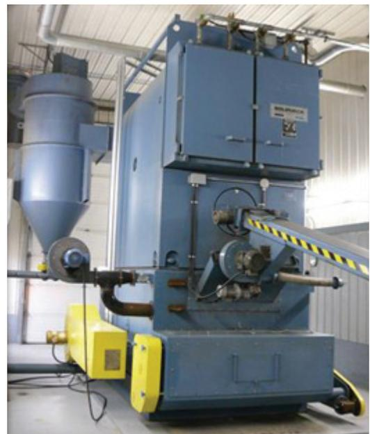
**Figure 3.** This wood-chip boiler's fully automated stoking system significantly reduces the daily labor required to maintain the system.
